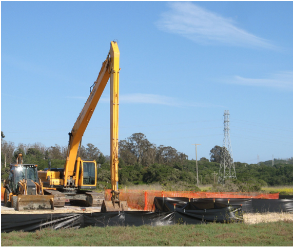
Photo P4.1 Black wildlife exclusion fencing to exclude sensitive amphibians. Orange fencing to preserve native plants. Photo: ESNERR
