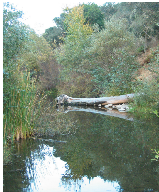
Photo P2.1 Large woody material placement using locally harvested trees.
