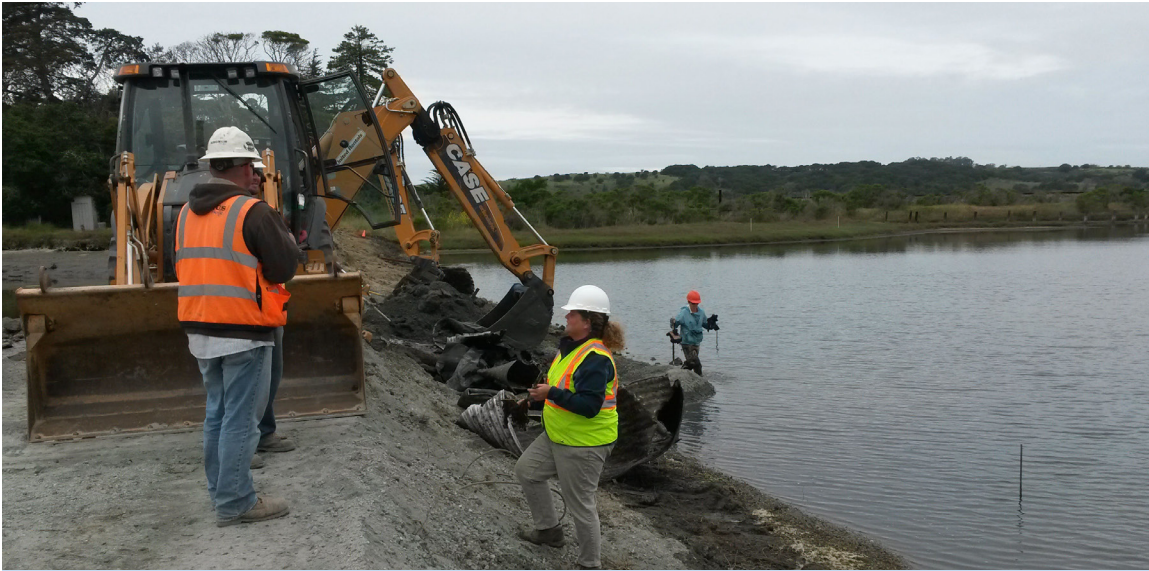
Photo PI.3 Installing culverts to improve water quality. Photo: ESNERR
