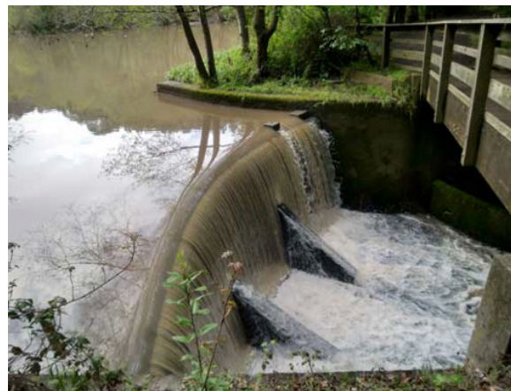
Photo P6.3 Spillway in use during flood
