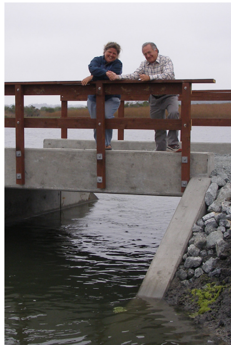
Photo P1.4 Improving tidal flow as part of a larger effort to improve water quality Photo: ESNERR
