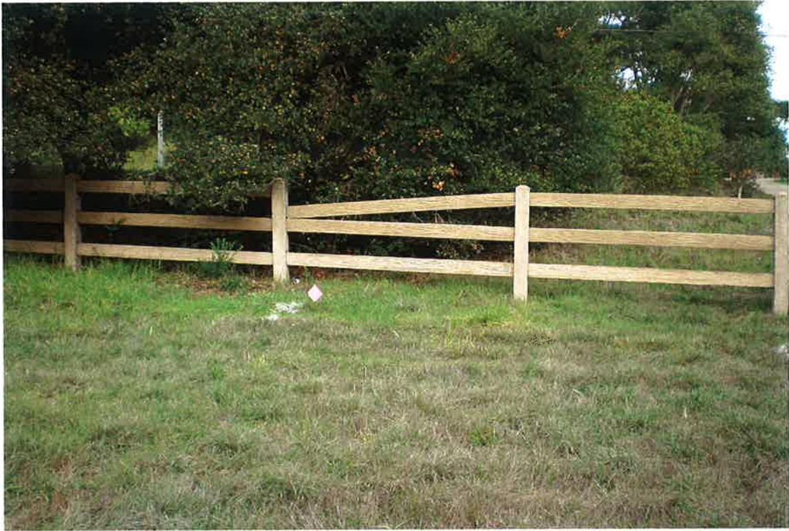
Figure 5. Broken Fence along Graham Hill Road (south of Deer Path Road).
