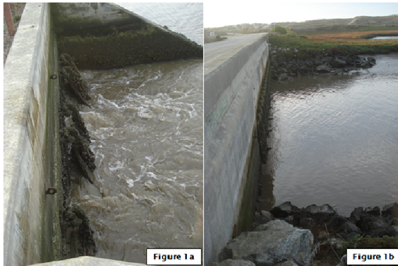
Figure 1. (a) Water flowing through the smaller section of three tide gates on the right bank of Potrero Road Bridge facing downstream (lower tide gates). (b) Downstream side of the main tide gates at low tide (November 5, 2010).
