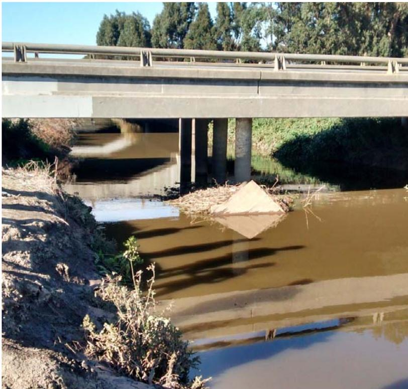
Figure C6: Haro St. bridge at the Haro St. sample site. Depth measurements were taken from the bridge at the second visible railing support from the left edge of the image.
