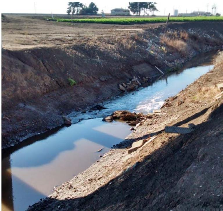
Figure C12: The Davis Rd. sample site. The hydraulic jump that separates the water quality and flow measurements was created by debris in the water channel.
