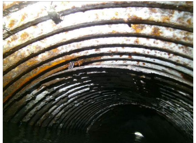
9. Pipe 3 CMP joints to RCP pipe, no leakage observed
