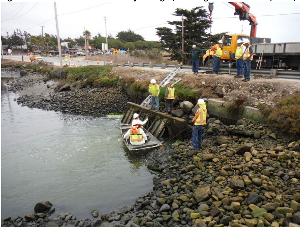
Figure 3. Culvert Outlets and Flap Gates; Initial Investigation with video camera in pipe (low tide 5pm October 9, 2014).
