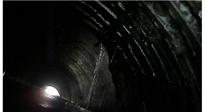
10. CMP to RCP joint in Pipe 1, minor leakage
