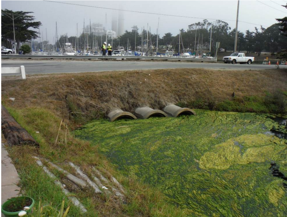
Figure 2. Culvert Inlets on Moro Cojo Slough (5.8 ft high tide October 8, 2014)
