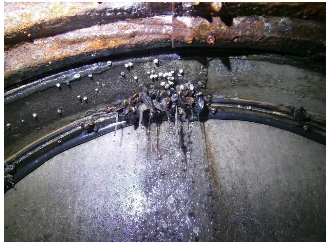
8. Pipe 3-Leakage from gasket, mussel fouling
