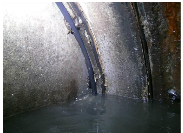
11. Tide Gate: Door, gasket, throat and headwall
