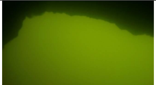
3.-Pipe 1-Left side of Hole in throat of gate
