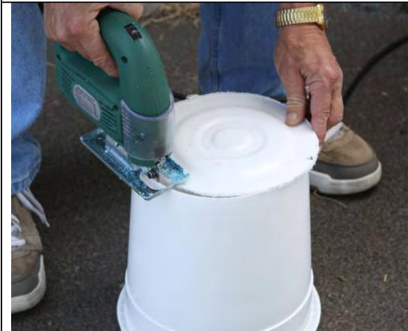
Figure 15. Use jigsaw to cut bottom out of one 2.5 gallon pail.
