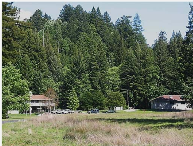
Little Basin Administration and Maintenance facilities
