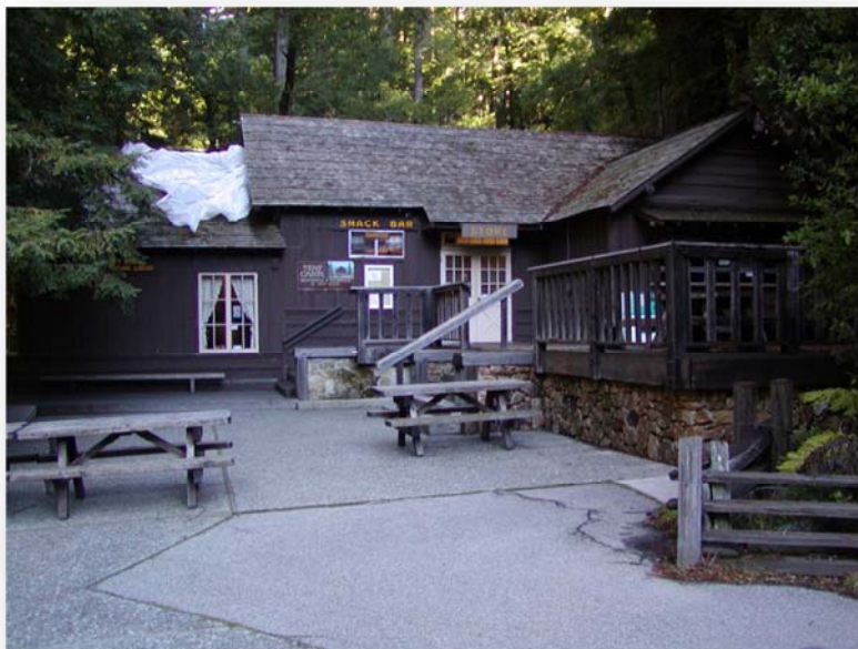
Nature lodge /Park store is one of several historic buildings in the park Headquarters area.
