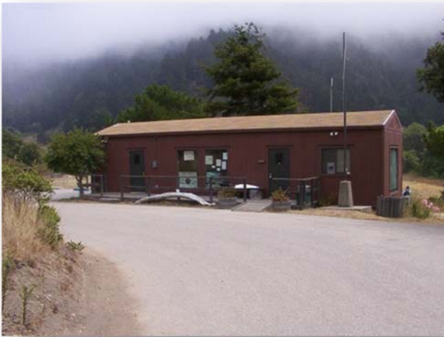
Existing Ranger office and interpretive facility
