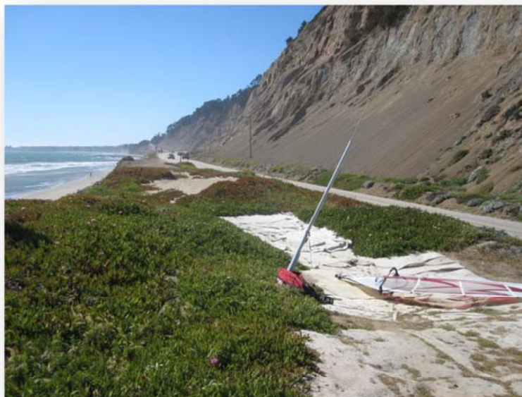
Highway 1 bluff erosion at Waddell Beach
