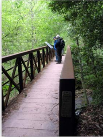
West Waddell Creek bridge on the Skyline to the Sea Trail
