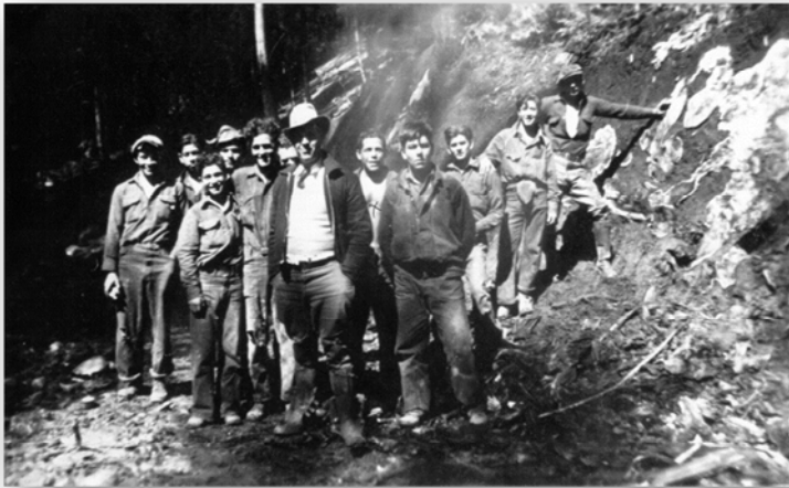
CCC men constructing a road
