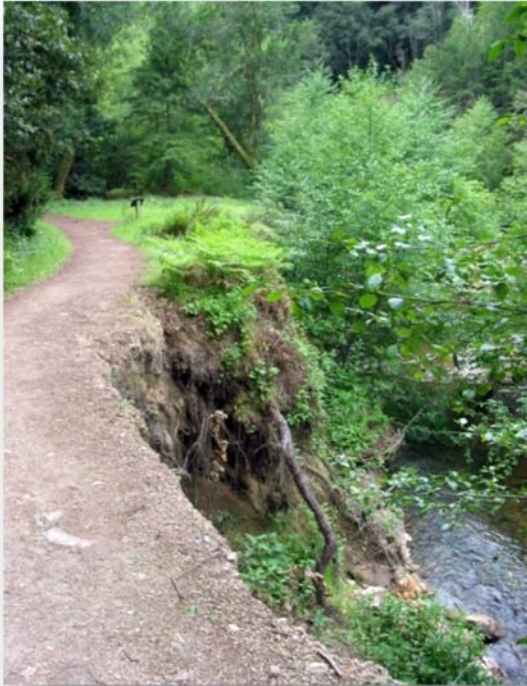
Creekside erosion along the Skyline to the Sea Trail
