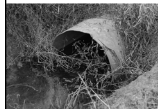
36 Inch Diameter Iron Culvert - Forming A Surface Connection Of South Tract Wetlands To North Tract – South Channel
