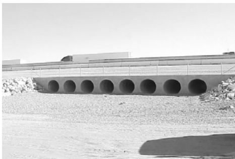
Finally it was agreed and decided among Caltrans, CDFG, and USFWS to place gravel within the rip raps of those culverts that had created a major threat.
