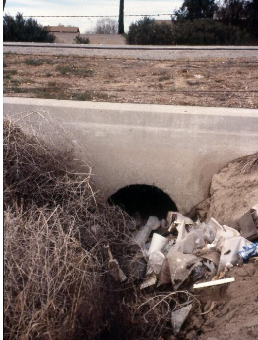
Figure 11. Drainage culvert under Highway 99 in Bakersfield, CA that was used as a den by San Joaquin kit fox.
