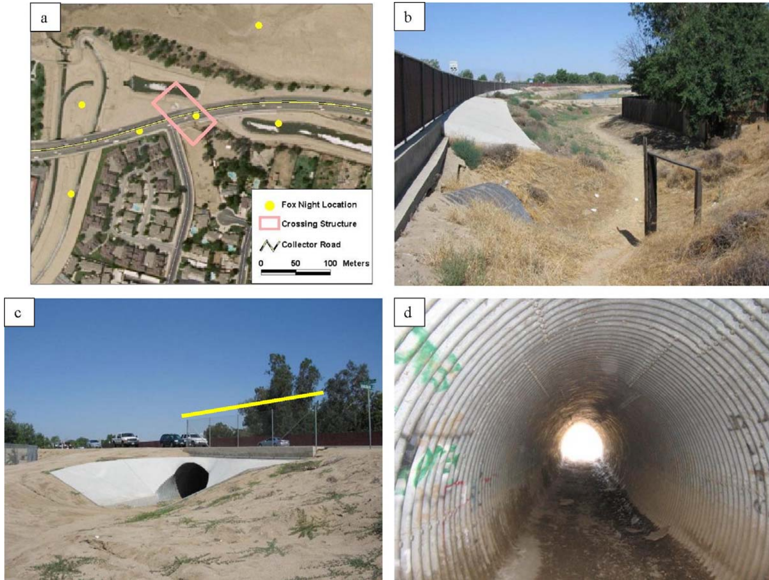
Figure 23. Truxtun Extension horse culvert, Bakersfield, CA. a) Aerial view of radio-tagged kit fox locations at horse culvert. b) View from pedestrian trail at south culvert entrance (canal in background). c) North culvert entrance. Yellow line depicts extent of fencing on north side of road. d) Culvert interior.
