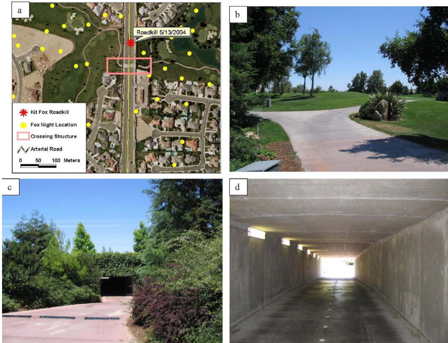
Figure 22. Buena Vista Road golf cart crossing structure, Bakersfield, CA. a) Aerial view of roadkill and radio-tagged kit fox locations at crossing structure. b) Habitat view from east entrance of crossing structure. c) Approach view to east entrance. d) Passage interior.
