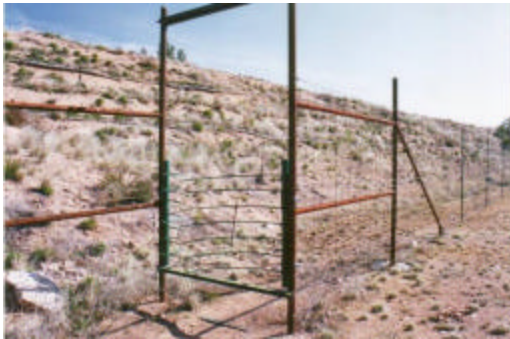
Figure 4-21. Ungulate fencing with 1-way gate (Arizona).
