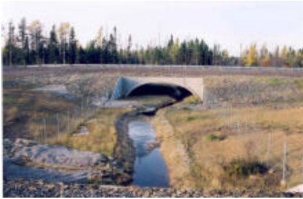
Figure 4-19. Wildlife fencing with arch culvert (New Brunswick).
