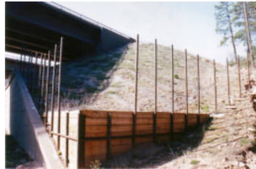
Figure 4-22. Ungulate fencing (2.5 m high) with 1.5 m high escape jump (Arizona).
