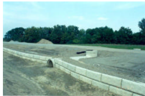
Figure 4-24. Bayview Avenue amphibian tunnel funnel fencing (interlocking retaining wall material) (York Region, Ontario).
