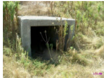
Figure 4-12. Concrete box culvert, Kitchener.
