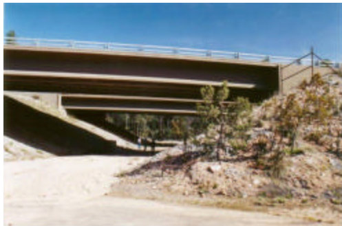
Figure 4-23. Ungulate underpass with fencing tied to structure (Arizona).
