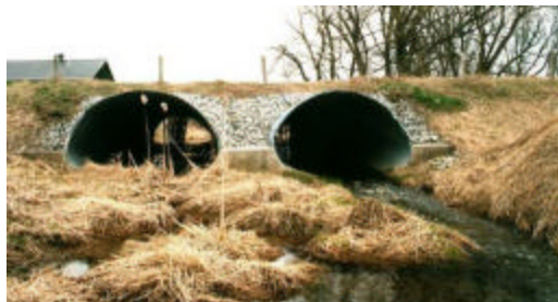
Figure 4-13. Open arch style culvert – Double cell.
