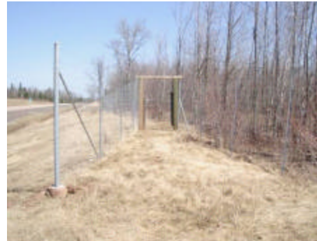
Figure 4-20. Frontal view of one-way deer gate with funneling fencing (New Brunswick).
