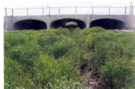
Figure 4-14. Multi-cell pre-cast open bottom culvert, Markham.
