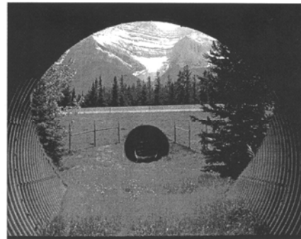
A culvert undercrossing, trans-Canada highway, Banff National Park; built in 1998
