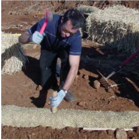
Installation of erosion control
