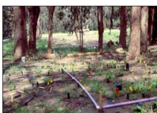
Drip-ring irrigation installation, Spring 2001
