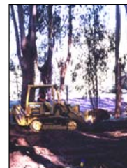
Heavy equipment removing duff layer, Fall 2000
